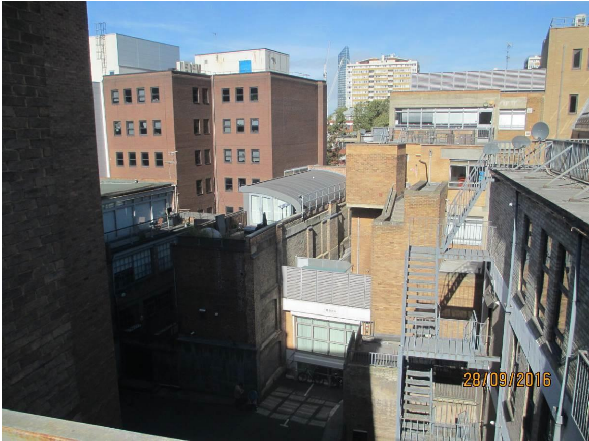
Image 6: View to rear from roof of application site
