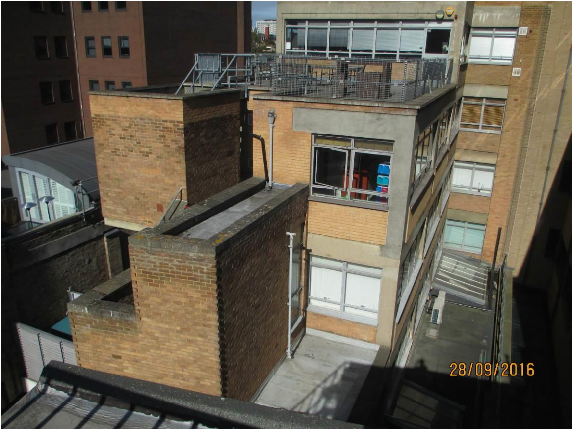
Image 4: Neighbouring property to rear (138-140 Old St) view from application site
